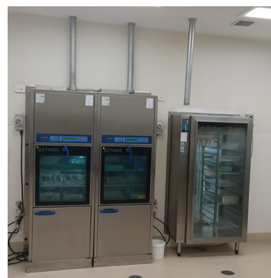
Figure 11 Existing Batch Washers & Pass-Through Cabinet
